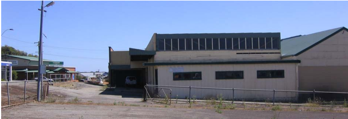
View looking North – the garage structure shall be demolished
