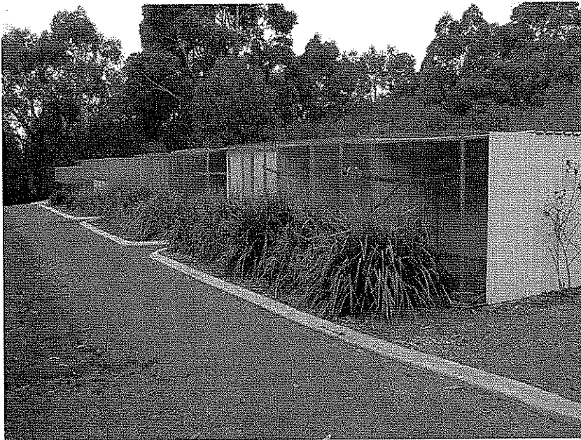
View of build quality and building material, landscaping and curb footpath
