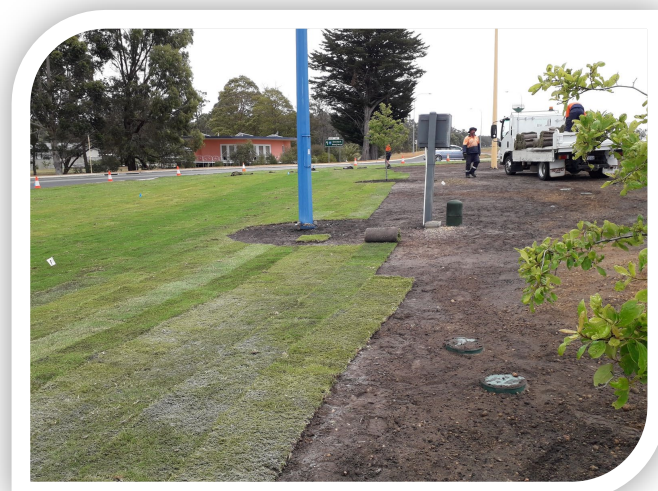
Laying of new reticulation and turf at the Albany Highway northern roundabout - November 2019
