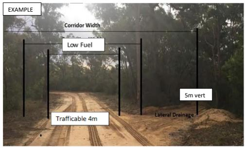
• Constructed to allow for appropriate drainage \* see drain types
