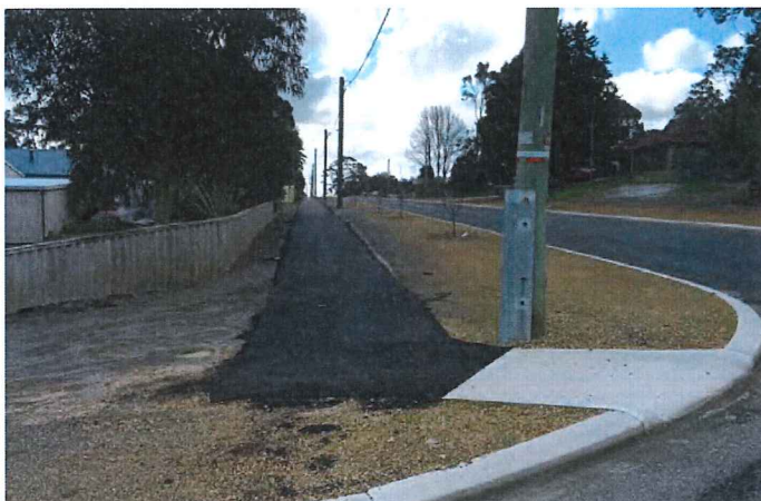
Photo 1: New asphalt path on Hassell Street
