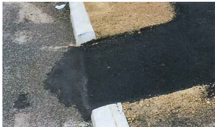
Photo 22: Asphalt Pram Ramp with vertical kerb cut (Hassell Street)
