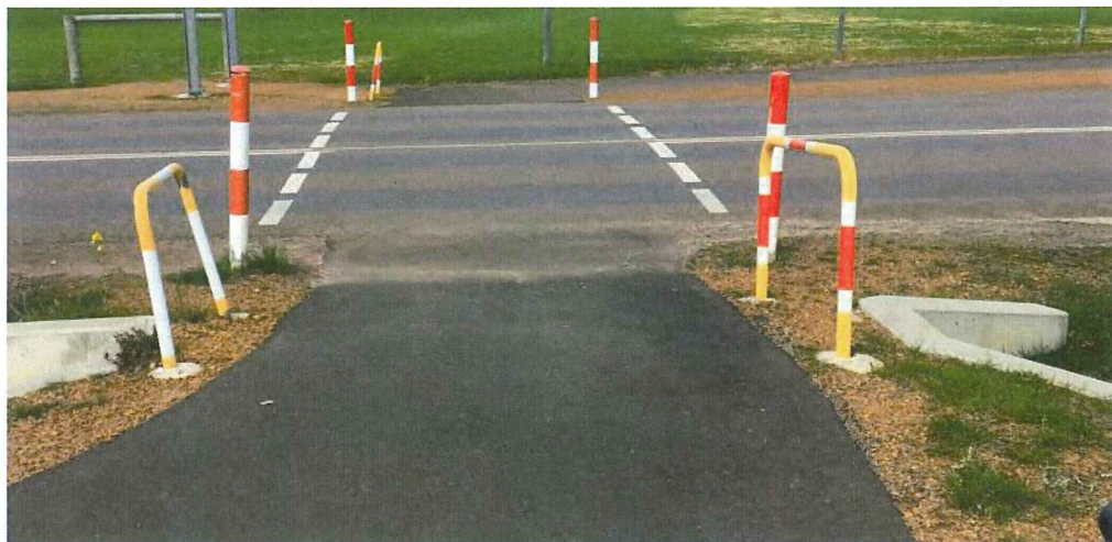
Photo 28: Crossing on Woogenelup Road with edge lining (as well as bollards and grab rails)
