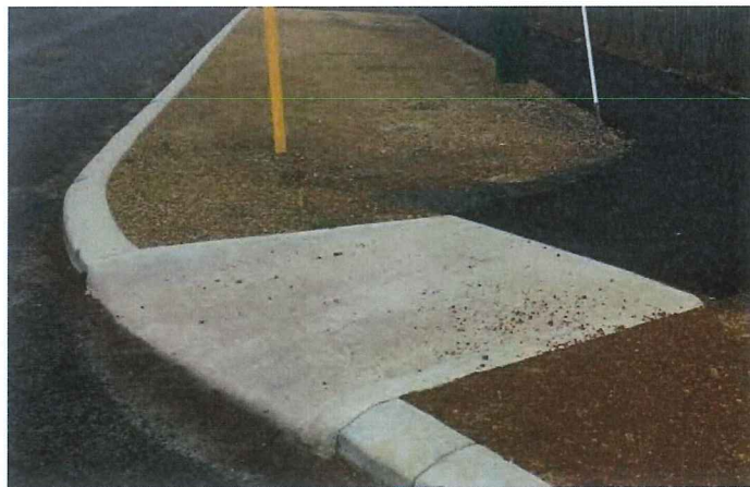
Photo 23: Concrete Pram Ramp constructed reasonably consistent with current standards (Hassell Street)
