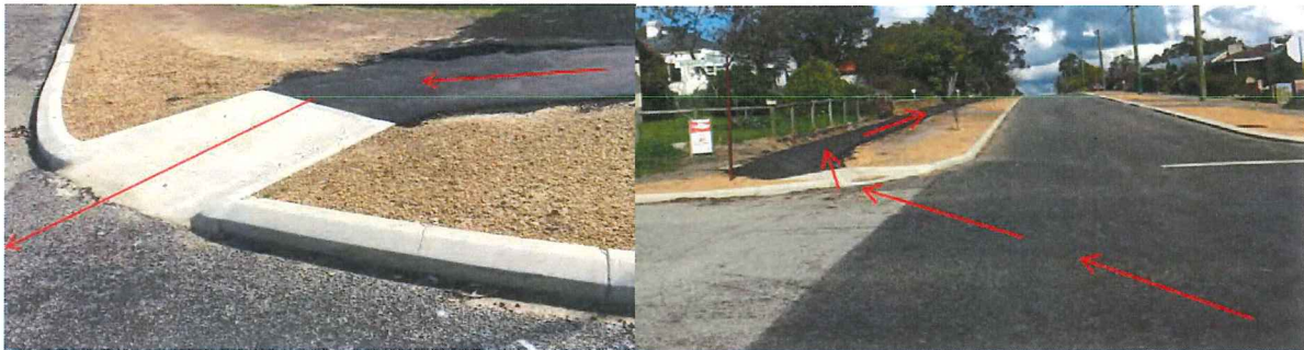
Photos 26 and 27: Pram Ramps at Hassell/Nunnarup Street intersection unsafely directing cyclist diagonally
