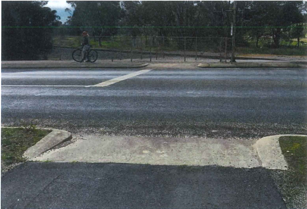
Photo 7: McDonald Avenue. Pram ramps
