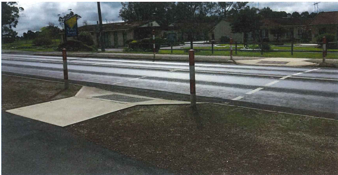
Photo 6: 460m south of Woogenelup Road. Bollards, concrete pram ramps with Tactile Ground Surface Indicators (TGS), edge delineation
