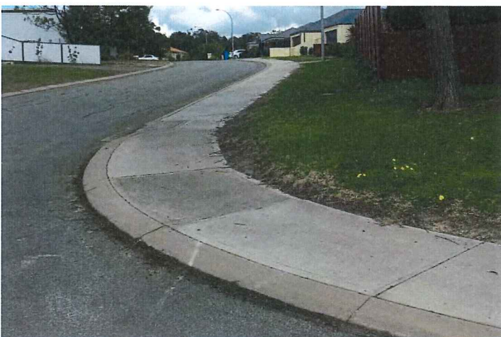
Photo 4: Concrete path on Donnelly Peak Place
