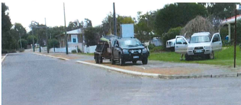
Photo 53: Hassell Street – no Pram Ramp at Haese Street
