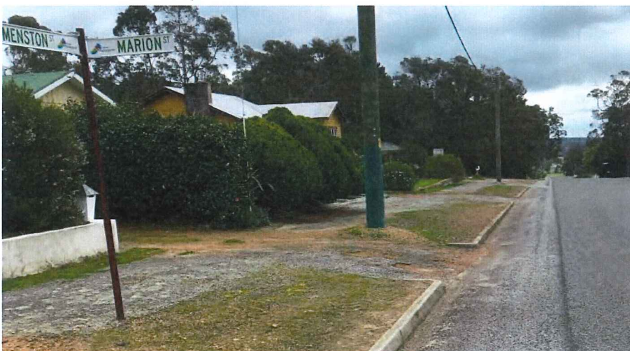
Photo 41: Menston Street asphalt overlay and pram ramps
