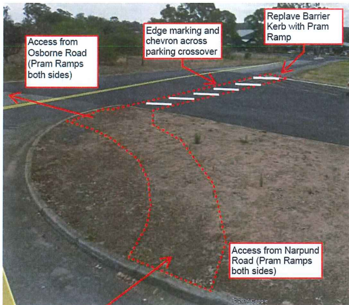
Photo 36: Narpund Road path upgrades at Osbourne Road intersection
