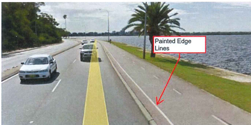
Photo 35: Edge Lining defining separation from behind kerb— Mounts Bay Road, Perth
