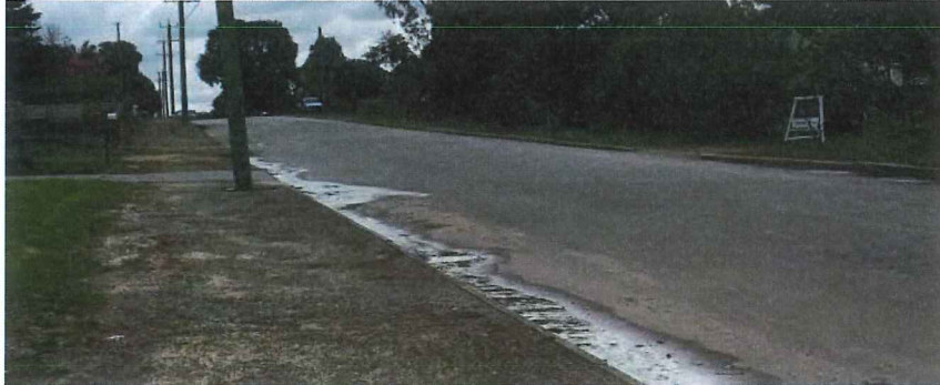
Photo 42: Mount Barker Road asphalt overlay
