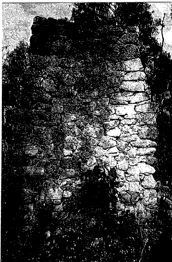
8/12/03 Stone fireplace and chimney of 'Moirs' hut' ruins from the north-east.
