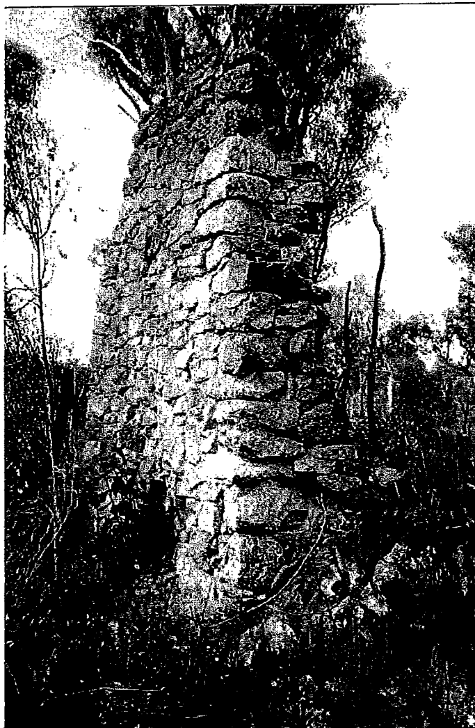
8/12/03 Stone fireplace and chimney of 'Moirs hut' ruins from the north.
