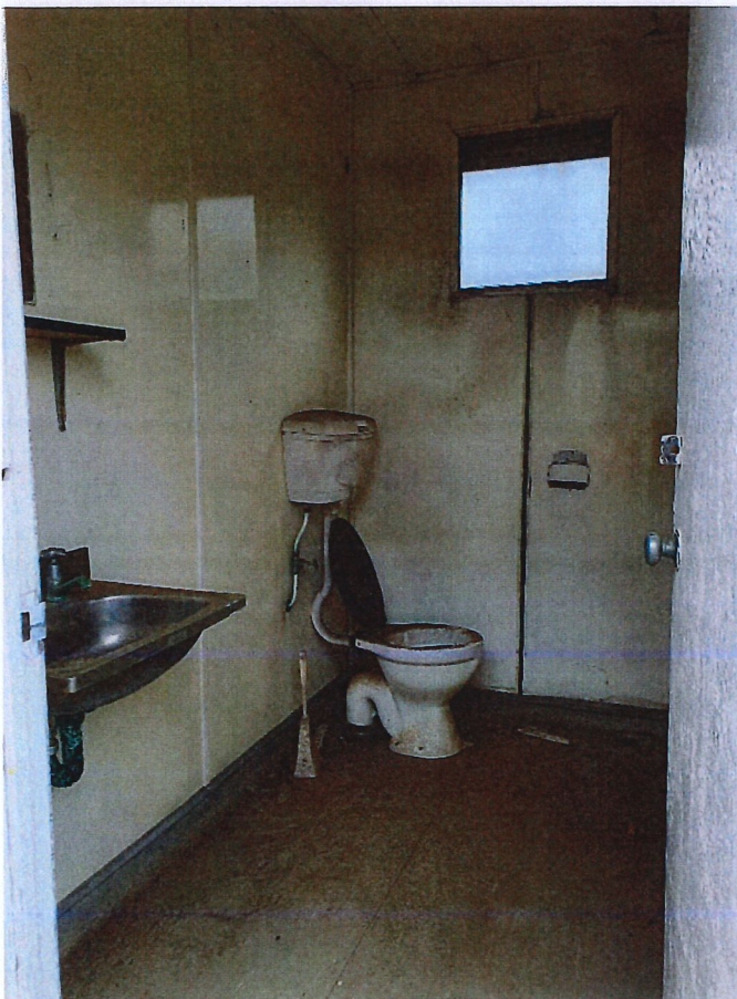
Demountable ablution block – no longer fit for purpose
