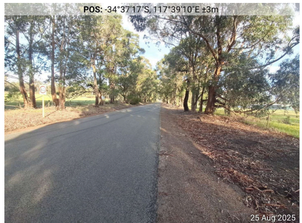
Photo: 16 Plot No: 8 Vegetation Type: Excluded 2.2.3.2(e) View east along McDonald Avenue with un-maintained verges with mixed forest ladder vegetation.
