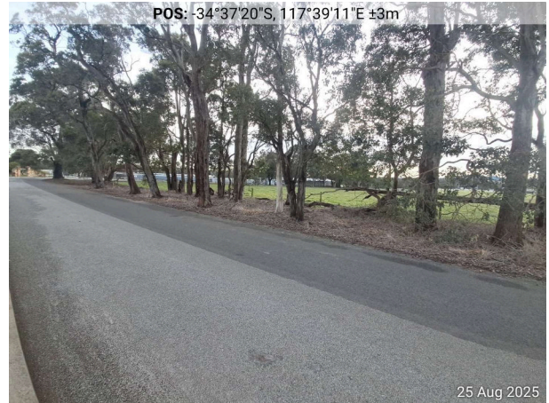
Photo: 20 Plot No: 8 Vegetation Type: Excluded 2.2.3.2(e) View north along Marmion Street with maintained verges of understory cleared tree line.
