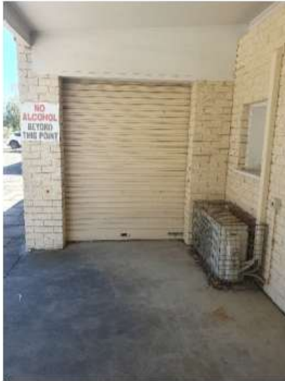
Roller Door Storeroom
