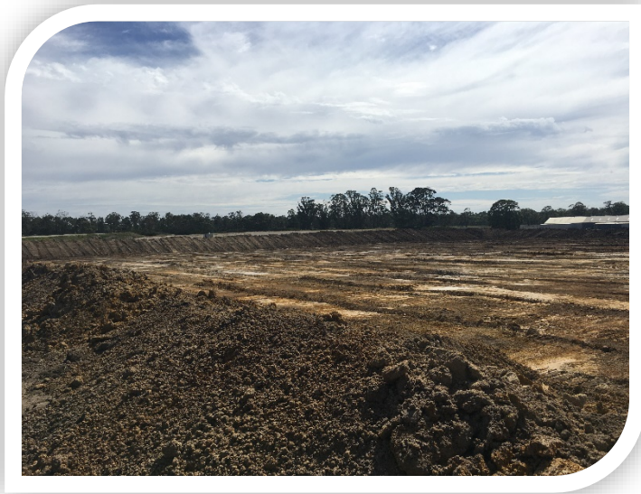
Construction of the 'turkey nest' dam in early 2021
