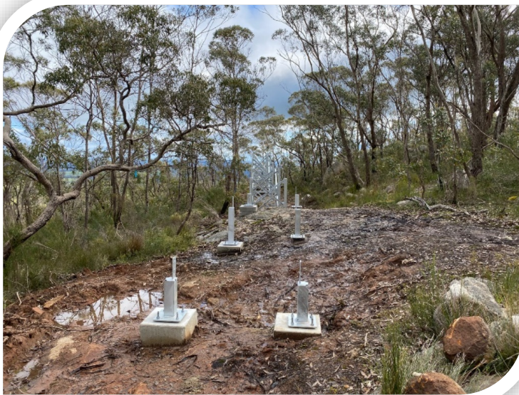
Mount Barker Hill boardwalk under construction
