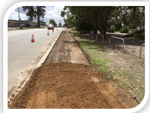
Preparation for dual-use footpath along section of Lowood Road, Mount Barker
