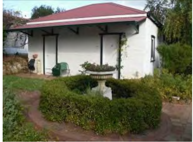
Photograph 4 – View of one of the accommodation quarters.
